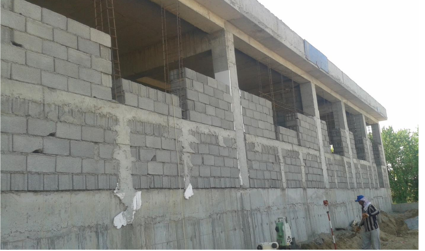
Akbugday TM Metal Clad Building while construction
